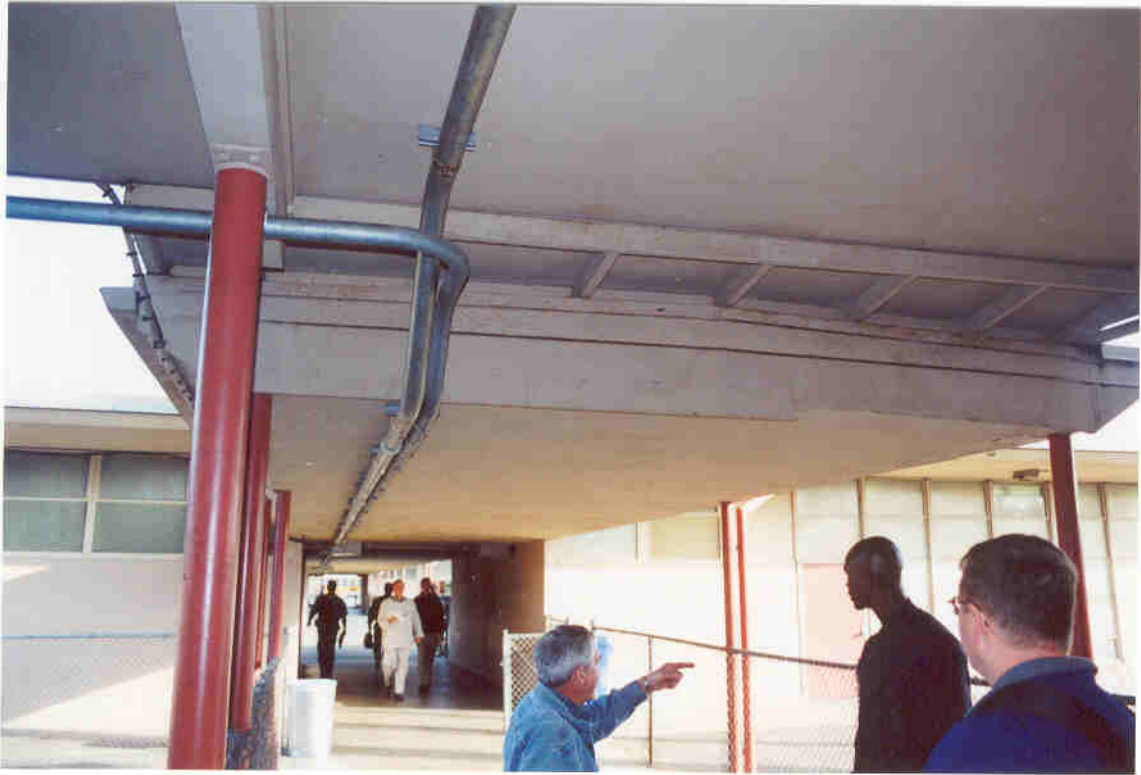
Figure 7: Electrical Conduits passing through covered walkways
