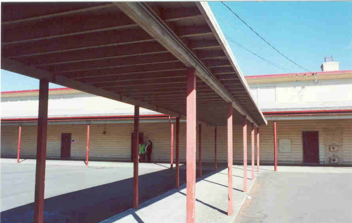
Figure 5: Covered Walkways at 1948 Classrooms
