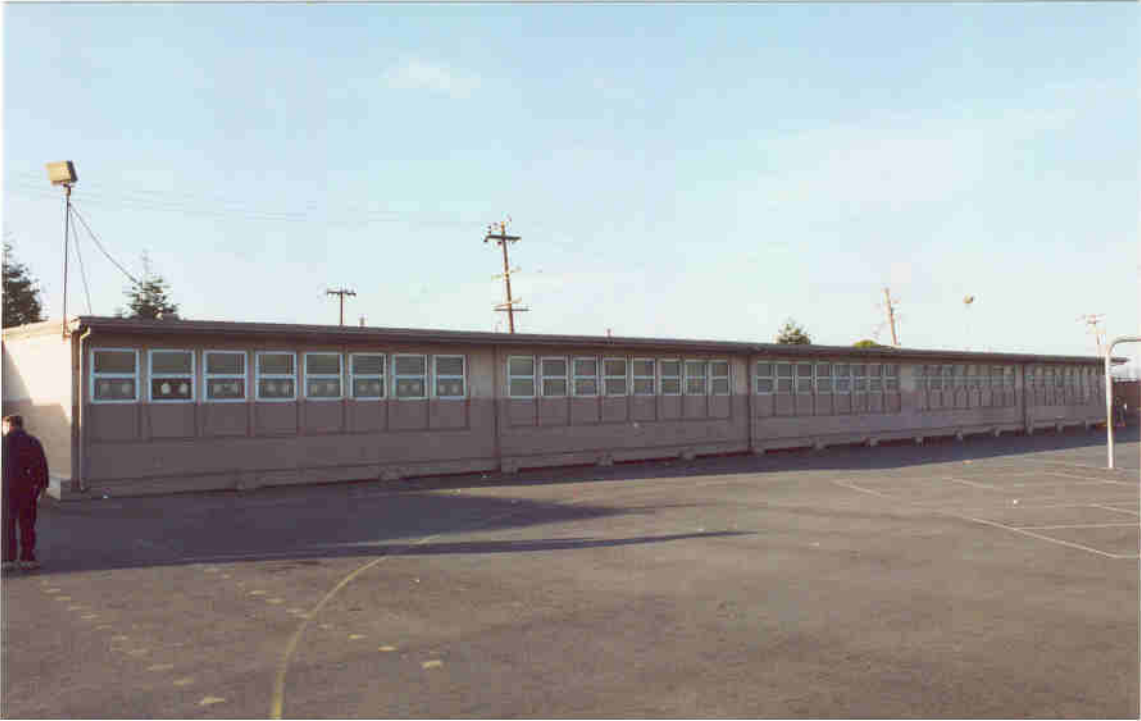
Figure 6: Classroom Building at south-west of site (1954) with intermittent foundations
